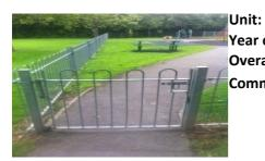
Fencing and Gates Year of Manufacture: Unknown **Overall condition:** Average Comments: Drop Pin Missing on Vehicle Access Gate 1 no post loose in ground, moss on fence and pedestrian gate. No padlock on the vehicle access gate
